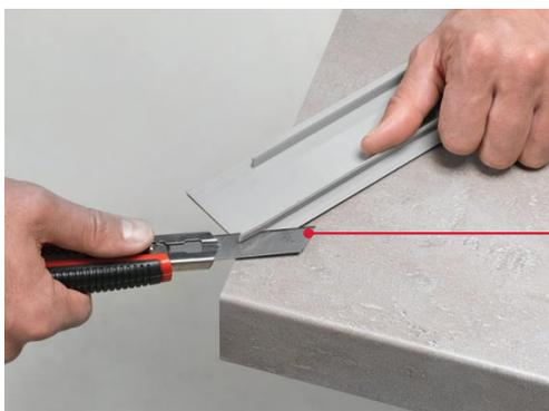
Cut out both sides of the ridge profiles with a utility knife, remaining pieces of the ridges should then be removed using a file
