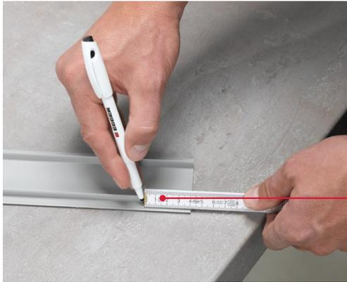
After the decor profile has been cut to size, the width of the frame in the worktop should be measured and marked.
