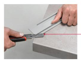
Cut out both sides of the ridge profiles with a utility knife, remaining pieces of the ridges should then be removed using a file
