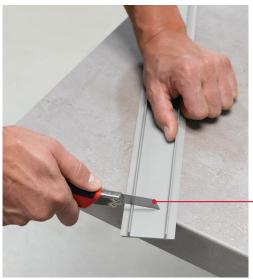
Make an incision on both sides of the ridge profiles - for example with a utility knife  $\,$
